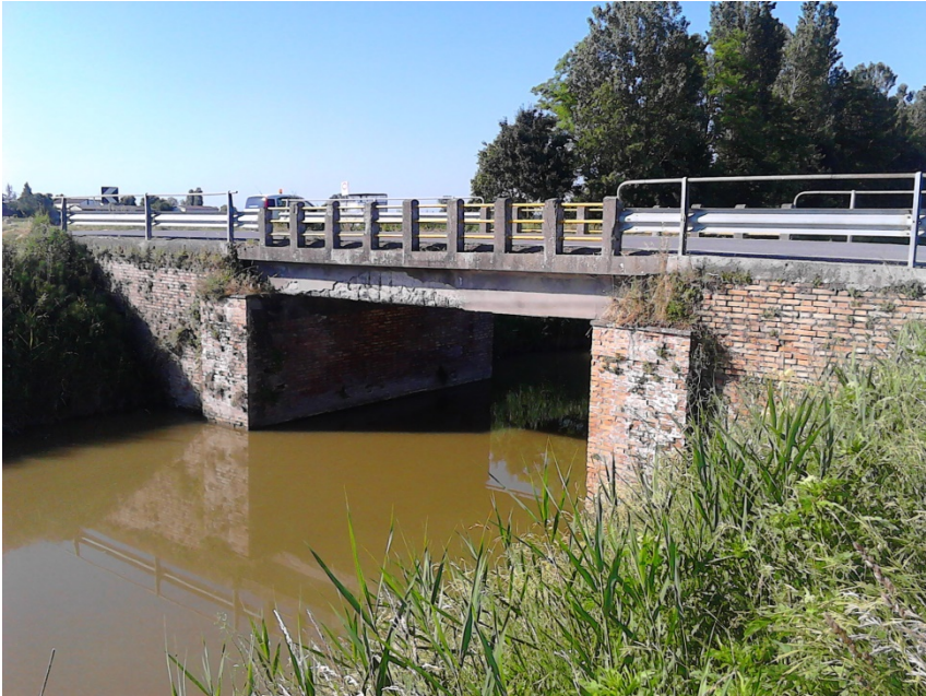
1. PONTE SP 105 PK 4+305 (Alfonsine)
