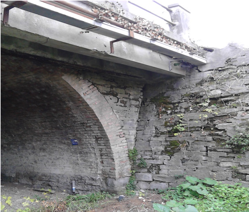
5. PONTE SP 302R PK 88+000 (Brisighella)
