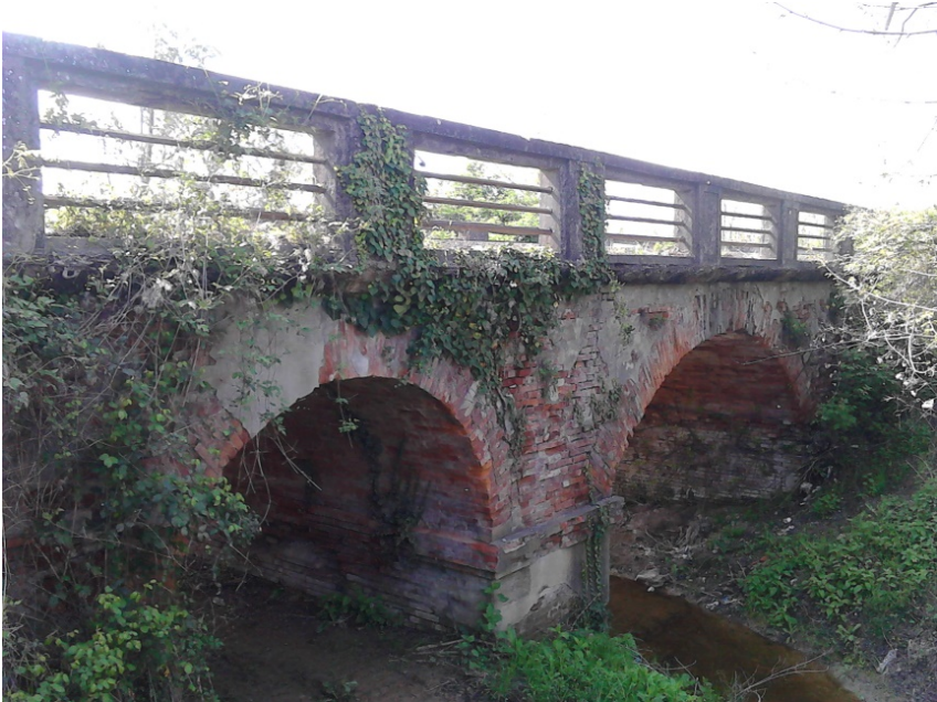
6. PONTE SP 302R PK 91+520 (Brisighella)
